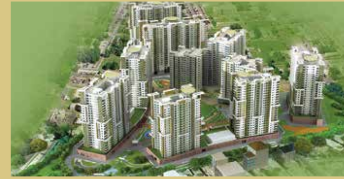
GREENAGE Hosur Main Road, Bengaluru
